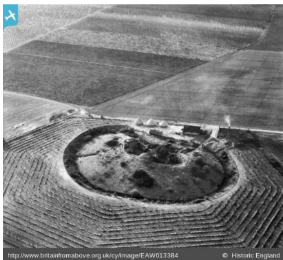
Figure 56. Fort Farningham 1948 (©Historic England)
