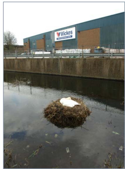
Figure 13. Concrete-lined River Darent, Dartford
