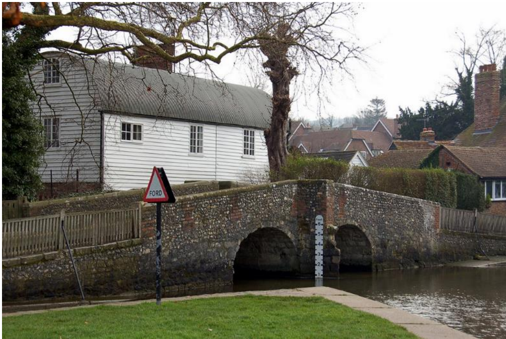
Figure 55. Eynsford Bridge (James Stringer Reproduced under a Creative Commons licence )
